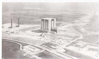
COMPLEX 39, Cape Kennedy, Fla. Vertical Assembly Building (center) is world's largest building, built by Army Engineers for NASA. Building is used to assemble and check out SA-TURN V/Apollo Space Craft for manned flight to the Moon. Crawler-transporter carries Saturn V/Apollo Špace Craft along crawler-way (right of VAB) to launch pad in upper right.
